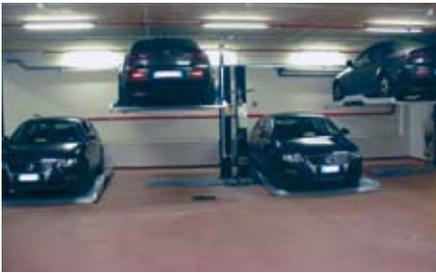
Sight of the garage basement. To avoid disturbing sights of electrical canalizations, the power supply of every single system has been realized through descents from the ceiling and the control panel has been installed directly on the column.
