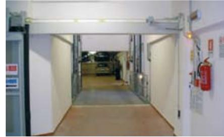
IdealPark car lift Mod. IP1-HMT V04 for the transport of the cars from the road to the underground garages. The system has been designed with special capacity of 3.500 kg suitable for the weight of the armored cars.
