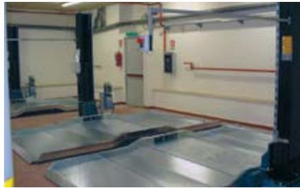
Sight of the systems without cars. The columns have been installed one on the right and one on the left to leave the space between the two systems free.
